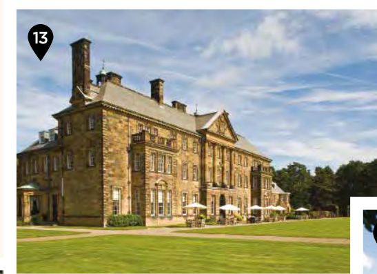
Crathorne Hall Hotel Yarm, North Yorkshire
